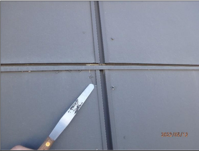
31. Overdriven fastener in fiber cement siding
