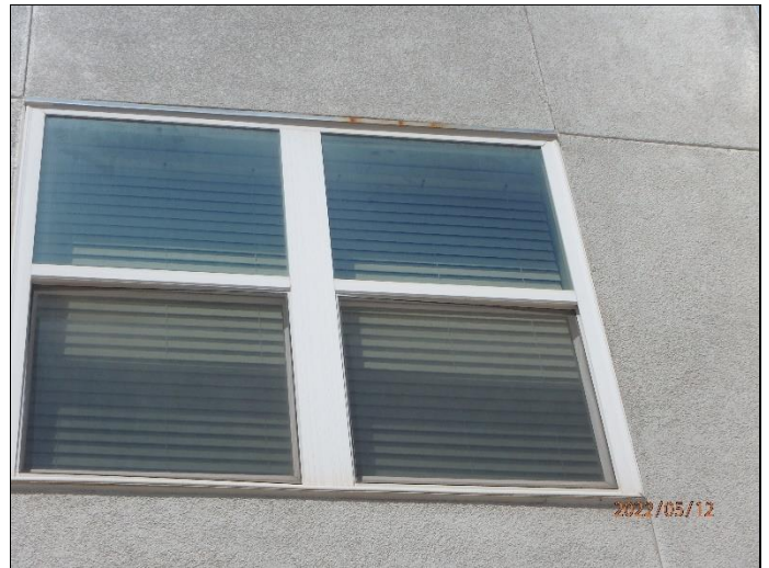
16. Corrosion at window head
