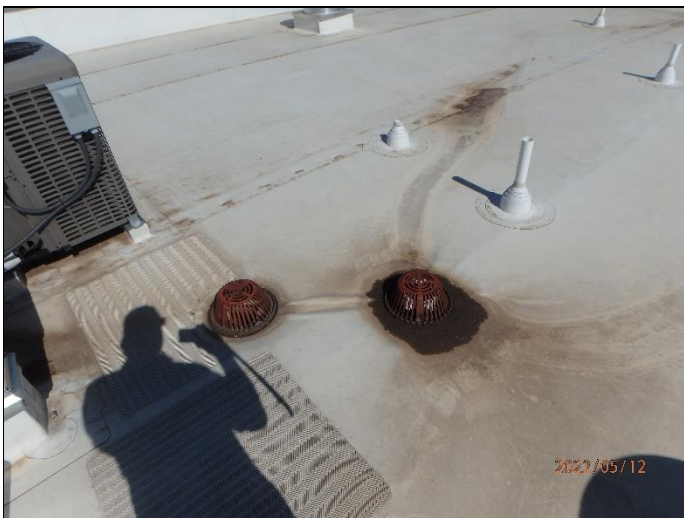
107. Primary and secondary drain – secondary drain is too high for drainage
