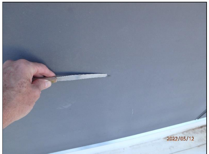
30. Overdriven fastener in fiber cement siding
