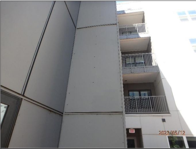
73. Overdriven fasteners in fiber cement siding
