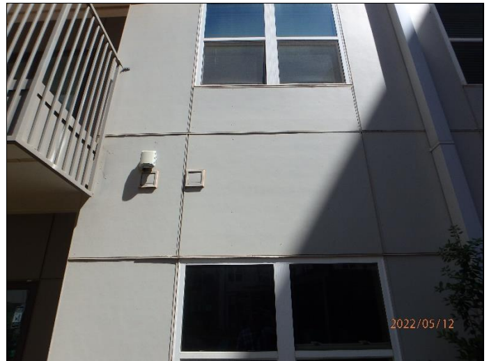
76. Overdriven fasteners in fiber cement siding
