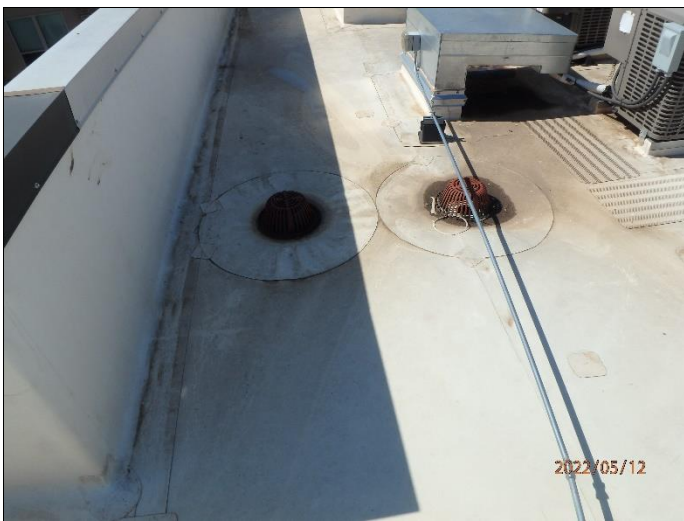
123. Primary and secondary drain – secondary drain is too high for drainage
