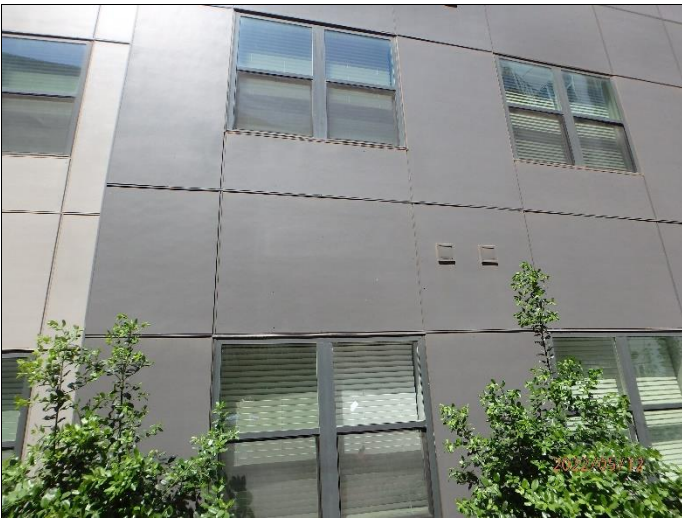
75. Overdriven fasteners in fiber cement siding
