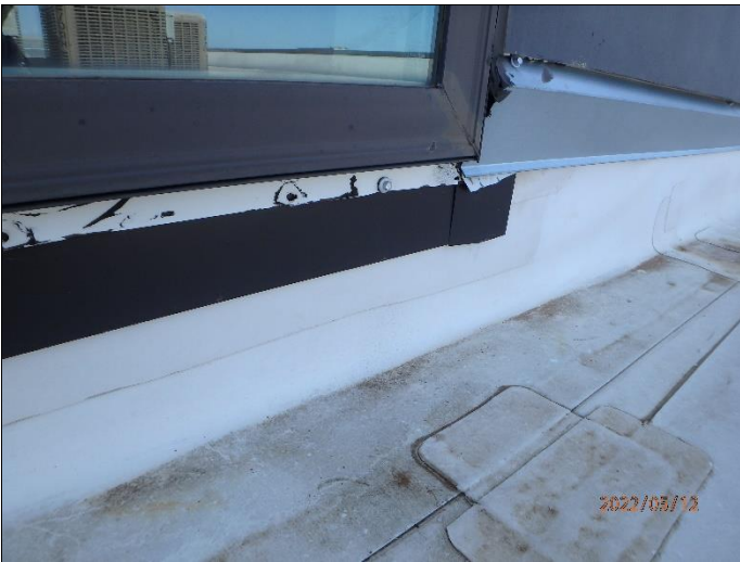
33. Missing counterflashing – Courtyard 1 roof
