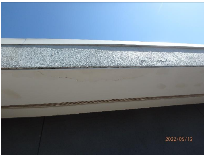
81. Deteriorated soffit
