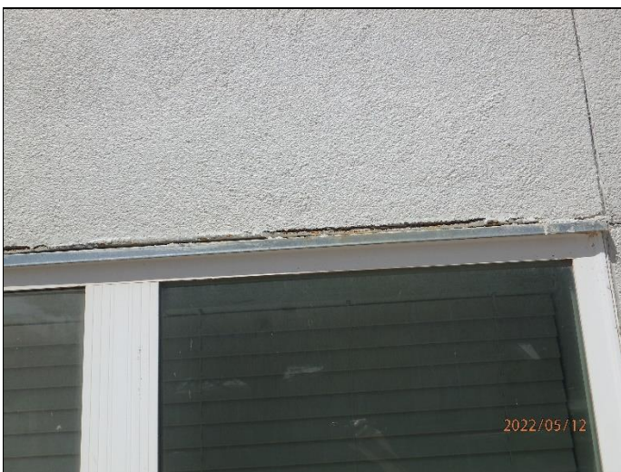
17. Corrosion at window head
