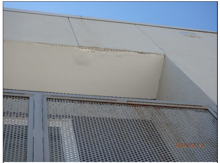
58. 5 th floor soffit deterioration
