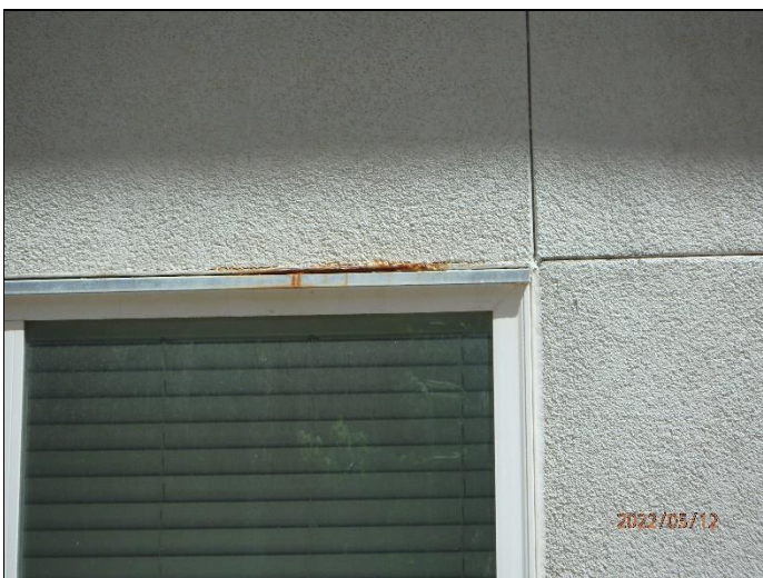
23. Corrosion at window head
