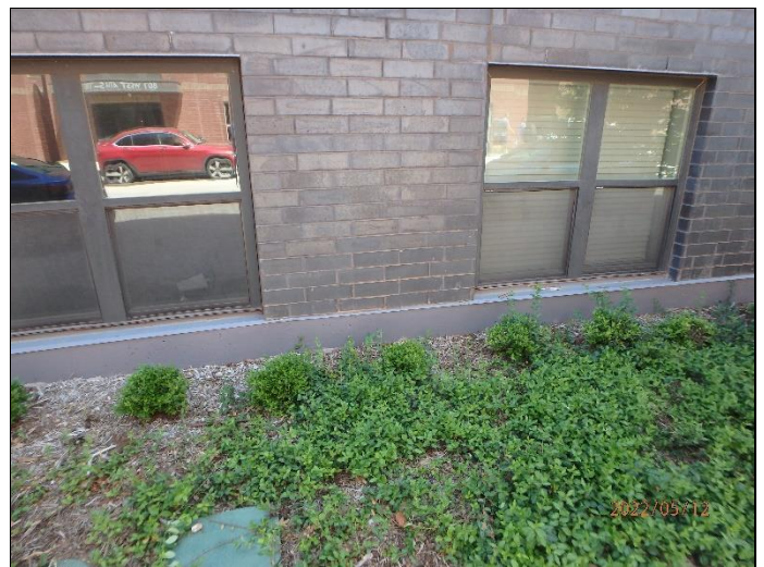
82. Missing weep vents
