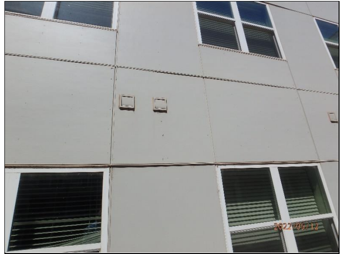
74. Overdriven fasteners in fiber cement siding
