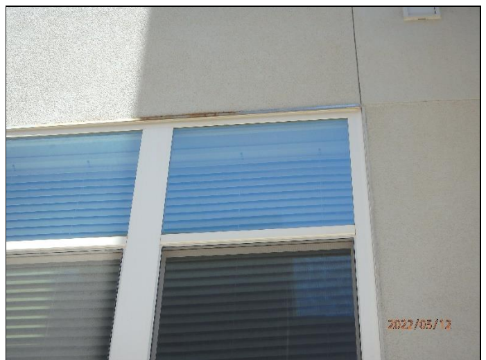
24. Corrosion at window head
