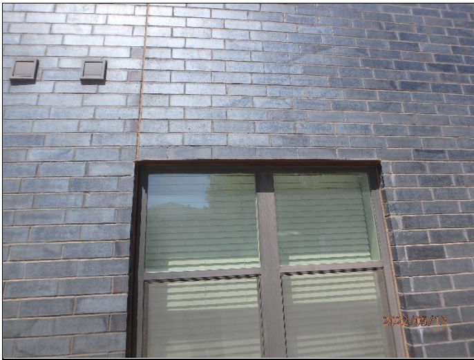
19. Head of window – missing weep vents
