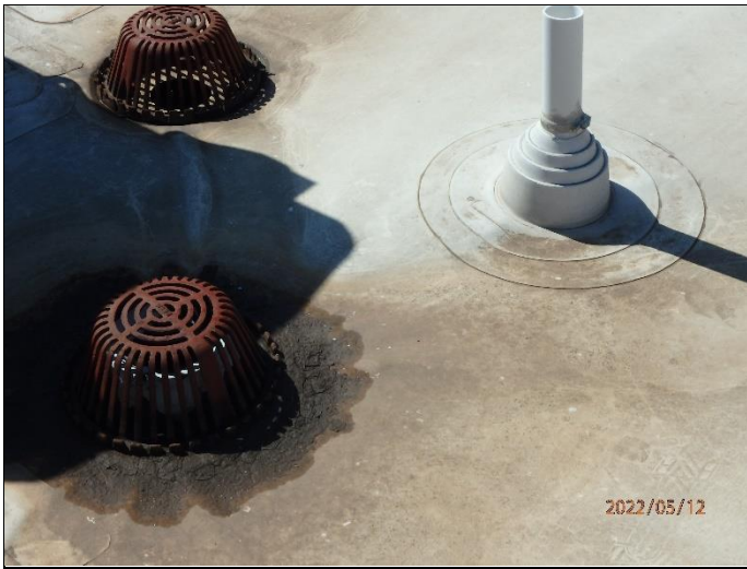
103. Primary and secondary drain – secondary drain is too high for drainage
