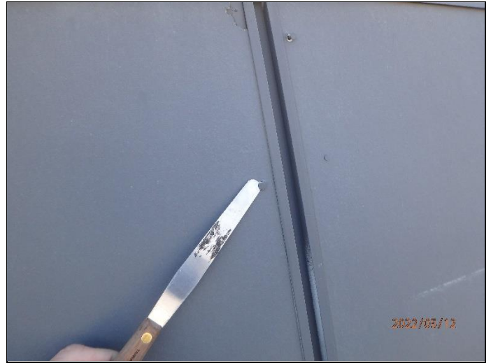
32. Overdriven fastener in fiber cement siding
