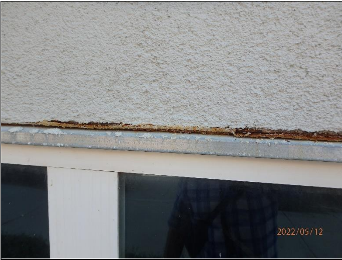
25. Corrosion at window head
