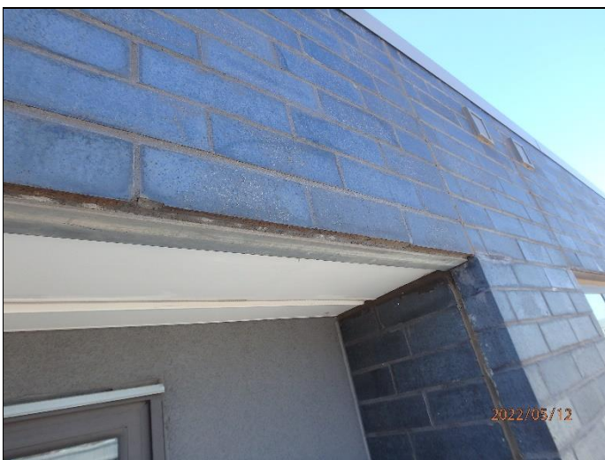
53. No weep vents above soffit, no drip
