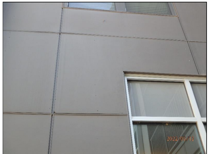
78. Overdriven fasteners in fiber cement siding
