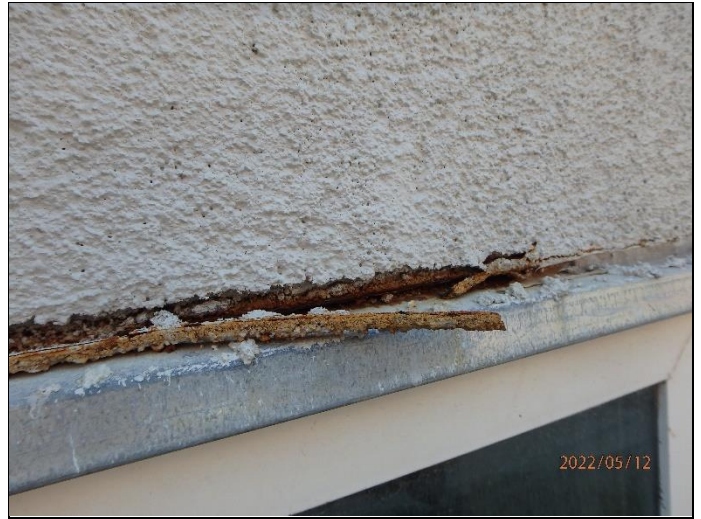
26. Corrosion at window head
