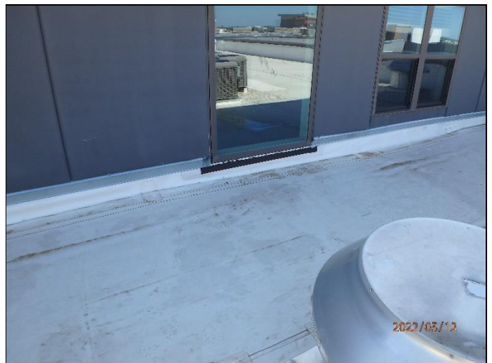
126. Missing counterflashing at base of window
