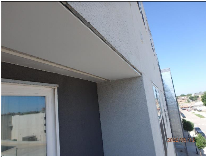
57. No drip at soffit
