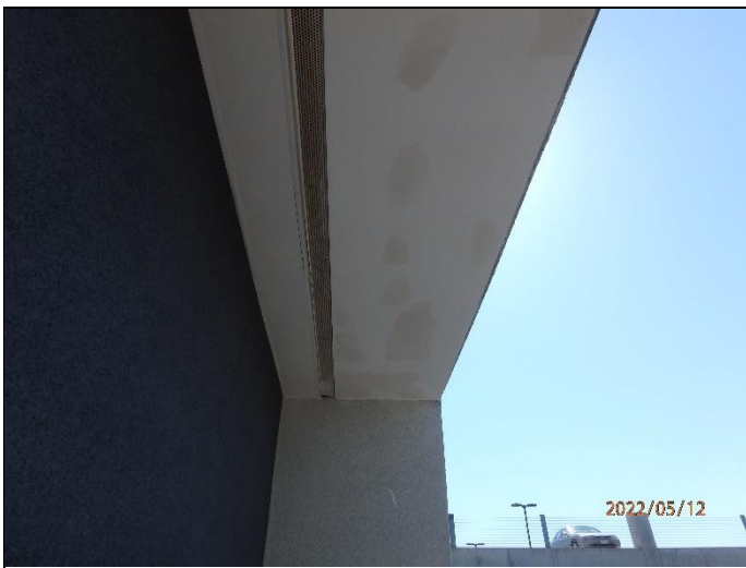
59. 5 th floor soffit deterioration
