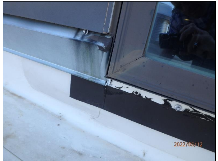
34. Missing counterflashing – Courtyard 1 roof
