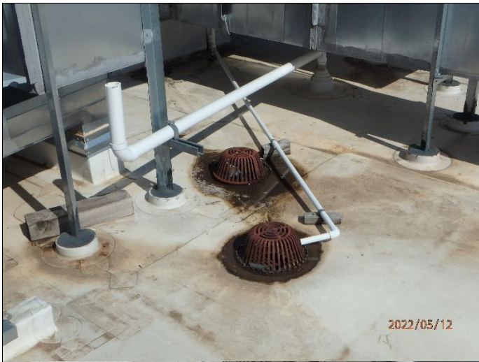
105. Primary and secondary drain – secondary drain is too high for drainage
