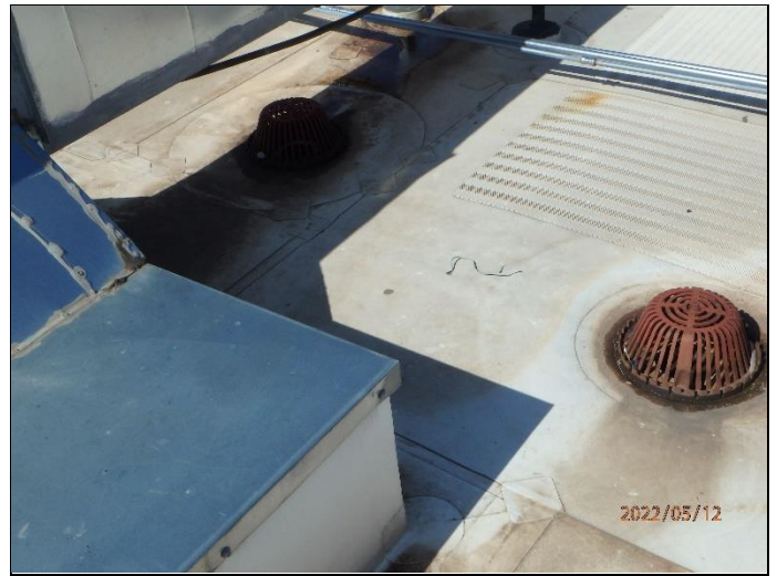
104. Primary and secondary drain – secondary drain is too high for drainage
