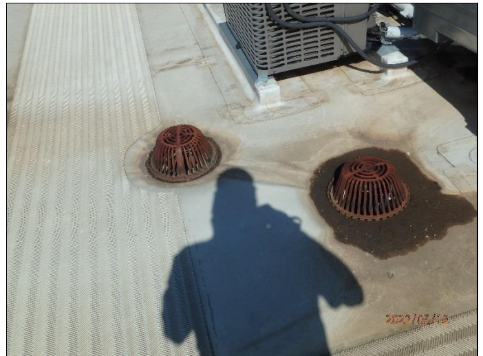
106. Primary and secondary drain – secondary drain is too high for drainage
