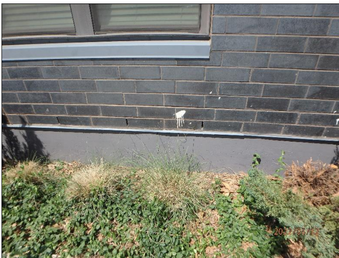
21. Base of face brick – missing weep vents
