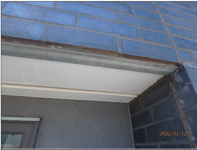
55. No weep vents above soffit, no drip
